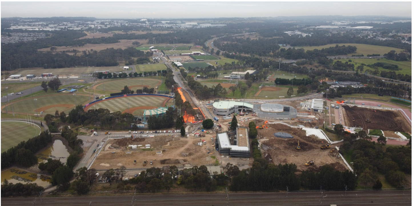
BEST Stage 1 – The BEST Hub – Constuction underway. Fully leased. Opening 2023.
